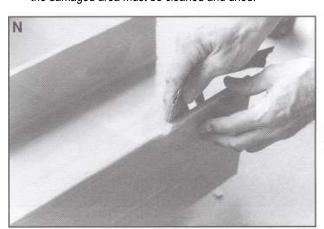
Epoxy or catalyzed resin may be used in this repair. If epoxy is used, the mixing procedure of the previous section is applicable. If catalyzed resin is used, mix 4 ounces of Hetron 92 with a few drops of DDM catalyst. (The exact ratio can be altered for ambient temperature). If so desired, milled fibre, Cab-o-Sil, or another filler may be added to improve the workability of the filling paste. Pigment can be added to match the colour of the section to be repaired.
