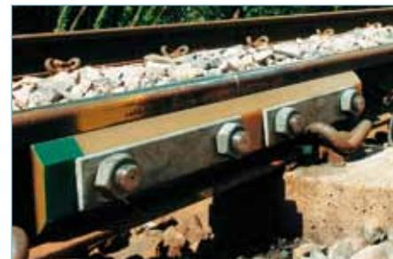
Special joints, as sample Emergency repair joints, distintively coloured for attention. Weight per joint appr. 20 kg.
